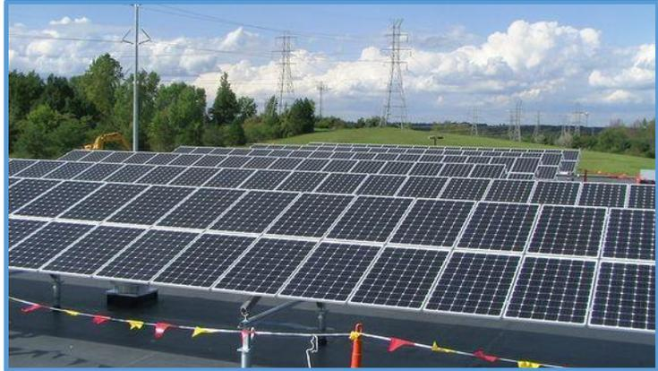
Michigan Solar Solutions installed a 95 kW solar array on a racking system integrated with the building structure during construction. As a result, Powers Distributing turned their roof into a source for 122.1 kWh per year of clean, green energy.
