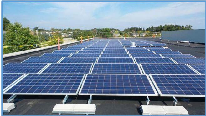
In Fall 2015, Michigan Solar Solutions installed a 75kW ballasted flat roof solar system at Controller Technologies offices in Detroit. The Controller Technologies system produces 86.5 kWh per year of clean, green energy.
