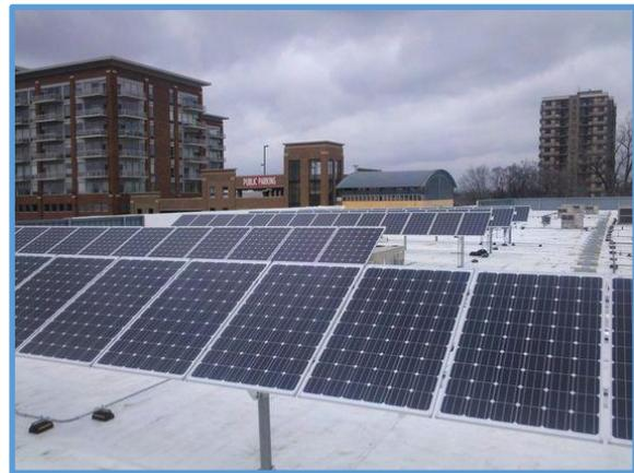
Michigan Solar Solutions installed a 40 kW solar array on a rooftop racking system integrated with the building structure. The Imagine solar system now produces 48.8 kWh per year of clean, green energy.
